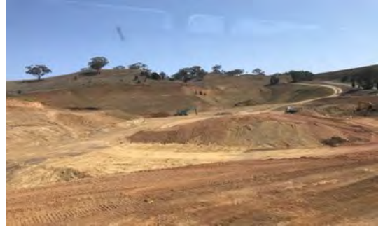
New Landfill site under construction
